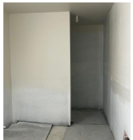
New Bathrooms with showers
